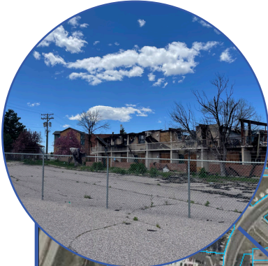
1. Deteriorated or Deteriorating Structures
