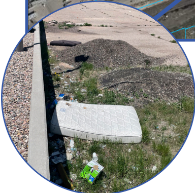
4. Unsanitary or Unsafe Conditions
