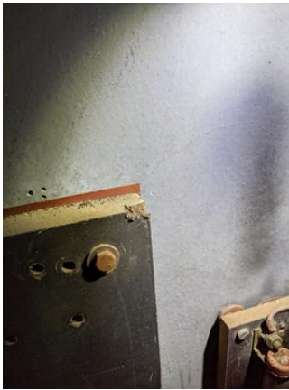
CHE-SP7077-170821-037 thru 039, 20% Asbestos, Gray fireboard
