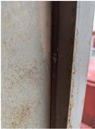
CHE-MP13835-130721-019 thru 021, 4.8% Asbestos, Gray door sealant
