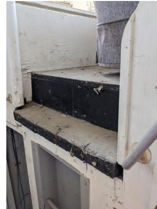
CHE-DRGW01481-160721-013 thru 015, Asbestos Not Detected, Black mastic
