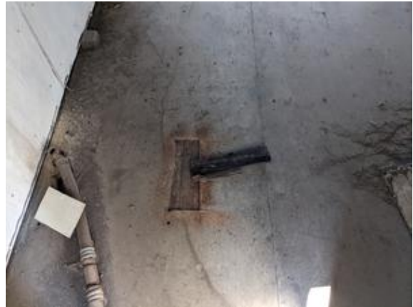
CHE-CNW11047-150721-004 thru 006, Asbestos Not Detected, Yellow mastic
