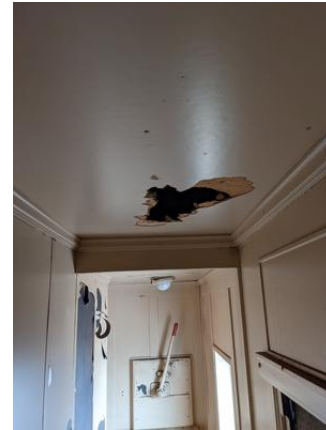
CHE-SP7078-180821-037 thru 039, Asbestos Not Detected, Masonite board (layered compound, mastic and fiberboard)
