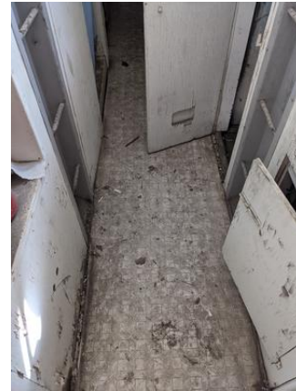
CHE-DRGW01486-160721-004 thru 006, Asbestos Not Detected, White sheet flooring and yellow mastic
