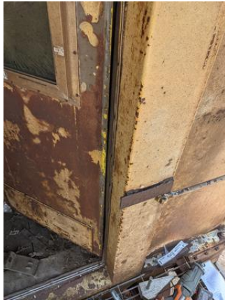
CHE-CN11097-140721-013 thru 015, Asbestos Not Detected, Black/brown caulk
