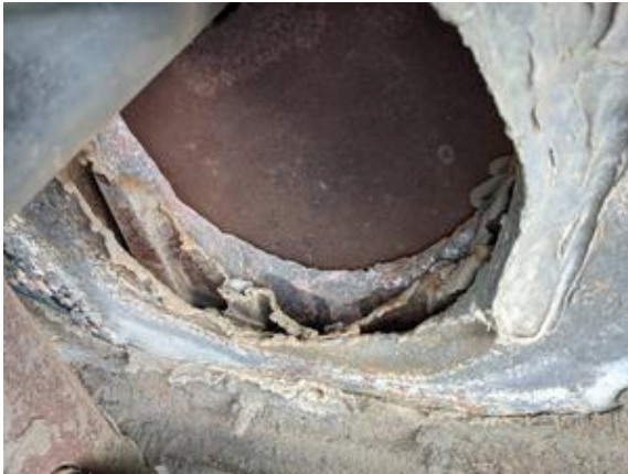
CHE-SP7077-170821-019 thru 021, 2.2% Asbestos, Gray sealant
