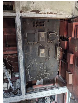
CHE-UP928-160821-007 thru 009, 40% Asbestos, Black Fireboard
