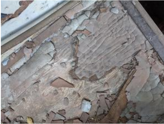
CHE-UP928-160821-037 thru 039, Asbestos Not Detected, Brown Vinyl Flooring (no mastic)
