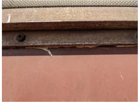
CHE-SP4641-130721-028 thru 030, 10% Asbestos, White window caulk
