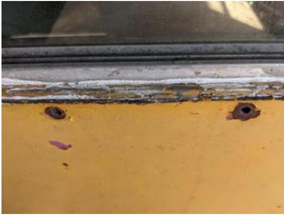
CHE-RI17017-150721-001 thru 003, Asbestos Not Detected, Silver coating
