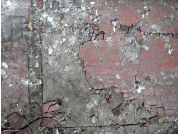
CHE-SP7078-180821-010 thru 012, Asbestos Not Detected, Red vinyl floor and brown mesh tape
