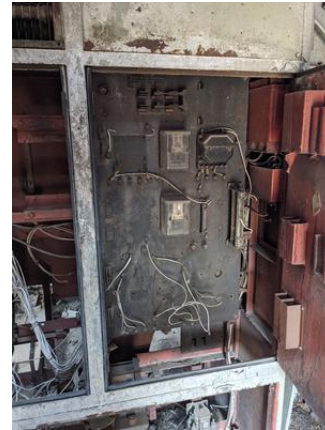
CHE-UP928-160821-004 thru 006, Asbestos Not Detected, White/black electrical wire wrap
