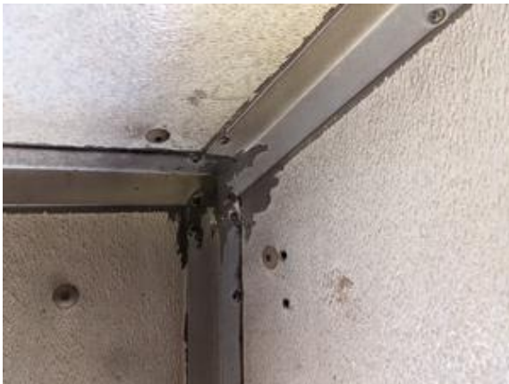
CHE-CNW11097-140721-004 thru 006, Asbestos Not Detected, White sealant
