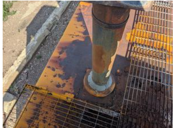
CHE-DRGW01476-170721-013 thru 015, 6% Asbestos, Black tar
