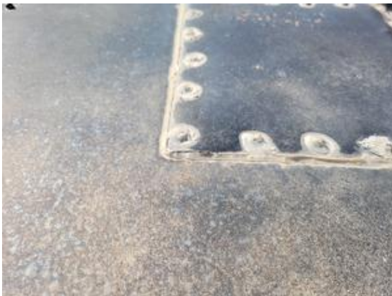
CHE-SP7077-170821-004 thru 006, Asbestos Not Detected, Clear silicone caulk
