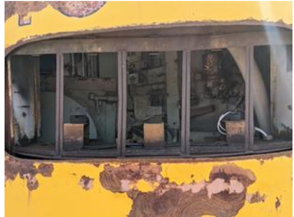
CHE-UP928-160821-022 thru 024, Asbestos Not Detected, Black Headlight Bulb Insulators
