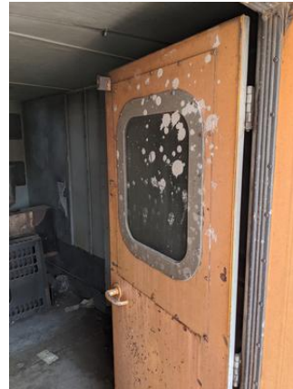
CHE-DRGW01524-170721-001P, PCB Not Detected, Black caulk
