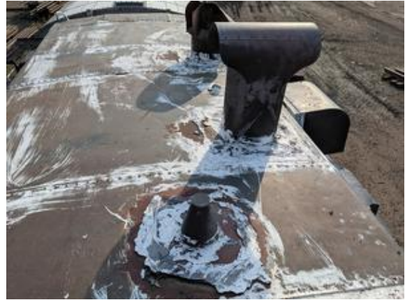
CHE-SP7078-180821-001 thru 003, 8% Asbestos, Black/gray sealant
