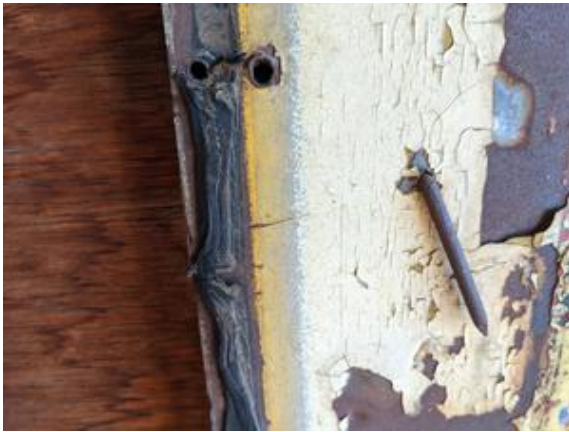
CHE-CNW11111-150721-010 thru 012, Asbestos Not Detected, Gray caulk
