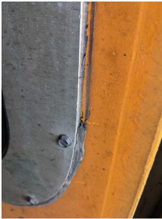
CHE-DRGW01489-150721-001P, PCB Not Detected, Black window caulk
