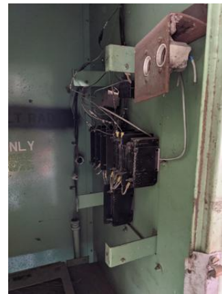
CHE-SP4641-130721-007 thru 009, Asbestos Not Detected, Black bakelite
