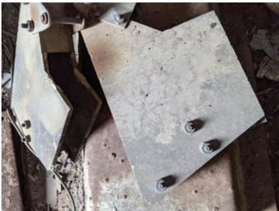
CHE-UP928-160821-025 thru 027, 20% Asbestos, Gray transite
