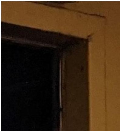
CHE-CNW11047-150721-001P, PCB Not Detected, Gray caulk
