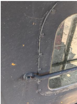
CHE-DRGW01486-160721-001P, PCB Not Detected, Black window caulk
