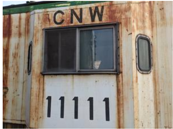
CHE-CNW11111-150721-002L, 5.1% Lead, Yellow
