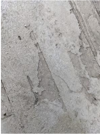
CHE-DRGW01476-170721-010 thru 012, Asbestos Not Detected, Black flooring and gray mastic
