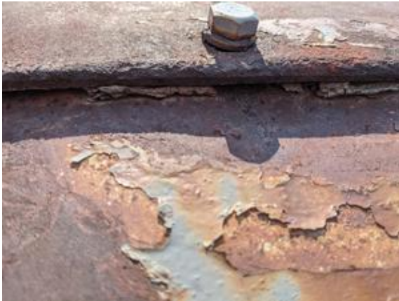
CHE-UP928-160821-031 thru 033, 10% Asbestos, Gray Coating
