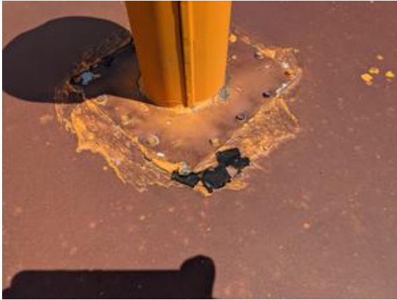
CHE-DRGW01489-150721-010 thru 012, Asbestos Not Detected, Black tar
