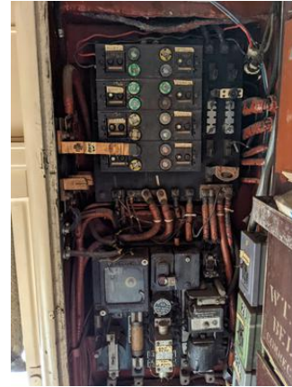
CHE-SP7078-180821-025 thru 027, 6% Asbestos, Black fiberboard
