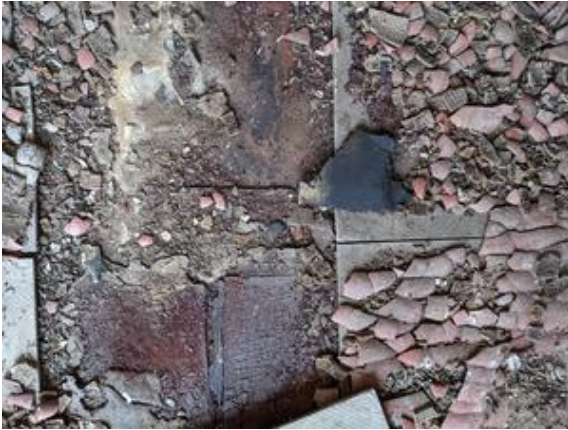
CHE-SP7078-180821-043 thru 045, 1.92% Asbestos, Red/black vinyl flooring
