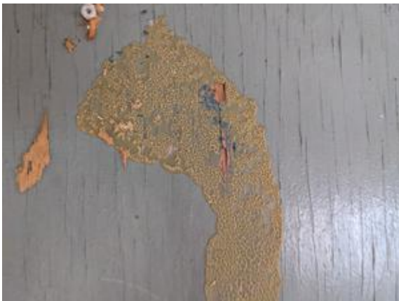
CHE-CNW11111-150721-007 thru 009, Asbestos Not Detected, Yellow mastic
