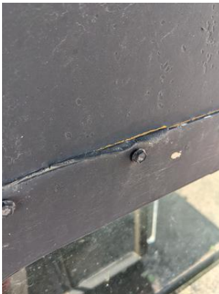
CHE-DRGW01481-160721-001P, PCB Not Detected, Black/brown window caulk
