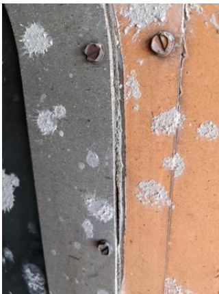
CHE-DRGW01524-170721-007 thru 009, 2% Asbestos, Black caulk
