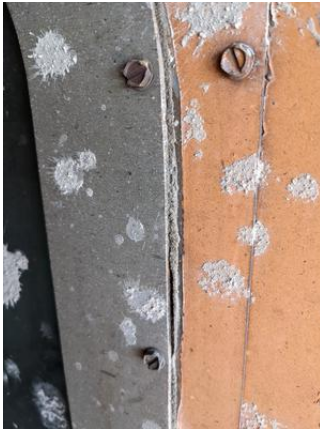
CHE-DRGW01524-170721-001P, PCB Not Detected, Black caulk
