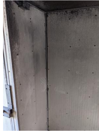
CHE-CNW11047-150721-001 thru 003, Asbestos Not Detected, Off-white sealant
