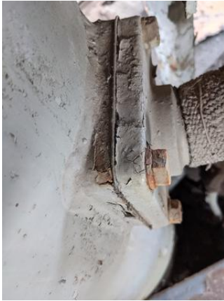
CHE-UP928-160821-028 thru 030, 30% Asbestos, Black gasket
