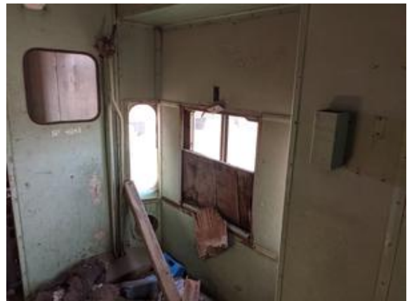
CHE-SP4641-130721-016 thru 018, 10% Asbestos, White window caulk
