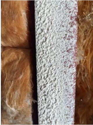
CHE-DRGW01524-170721-019 thru 021, 4.7% Asbestos, White coating
