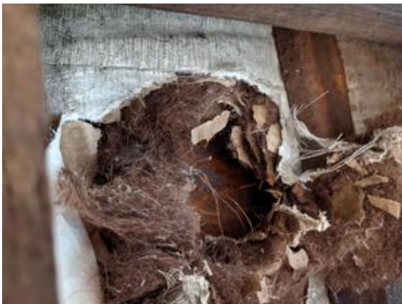
CHE-SP7078-180821-007 thru 009, 15% Asbestos, White/brown paper insulation
