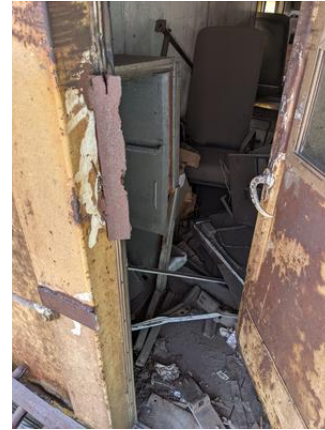
CHE-CNW11097-140721-001P, PCB Not Detected, Black/brown caulk
