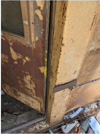
CHE-CNW11097-140721-001P, PCB Not Detected, Black/brown caulk
