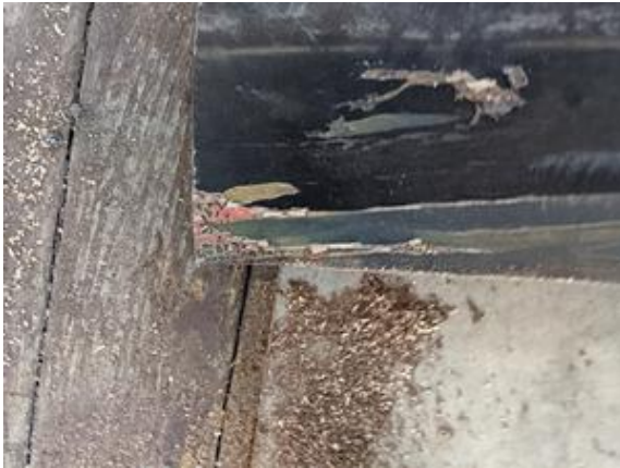
CHE-CNW11047-150721-004 thru 006, Asbestos Not Detected, Yellow mastic
