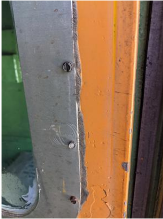
CHE-DRGW01476-170721-001P, PCB Not Detected, Gray/black window caulk
