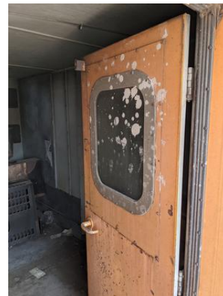
CHE-DRGW01524-170721-007 thru 009, 2% Asbestos, Black caulk
