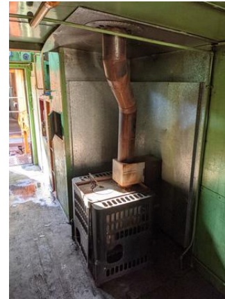
CHE-DRGW01476-170721-004 thru 006, Asbestos Not Detected, Brown fiberboard
