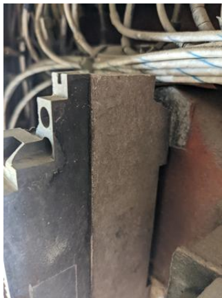
CHE-UP928-160821-016 thru 018, Asbestos Not Detected, Gray Bakelite
