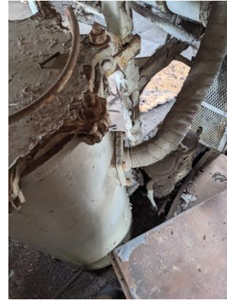
CHE-UP928-160821-028 thru 030, 30% Asbestos, Black gasket
