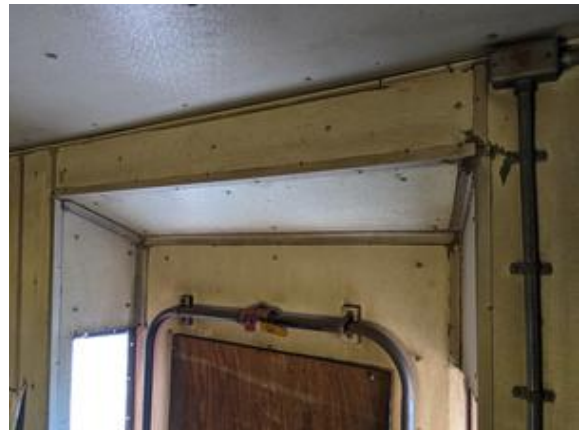
CHE-CNW11097-140721-004 thru 006, Asbestos Not Detected, White sealant
