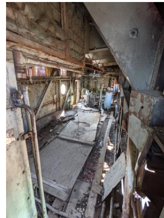
View of interior of railcar
