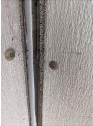
CHE-CNW11047-150721-001 thru 003, Asbestos Not Detected, Off-white sealant
