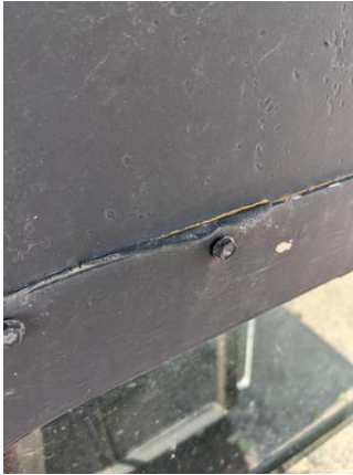
CHE-DRGW01481-160721-001 thru 003, Asbestos Not Detected, Black/brown window caulk
