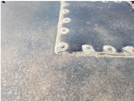
CHE-SP7077-170821-001P, PCB Not Detected, Clear silicone caulk
