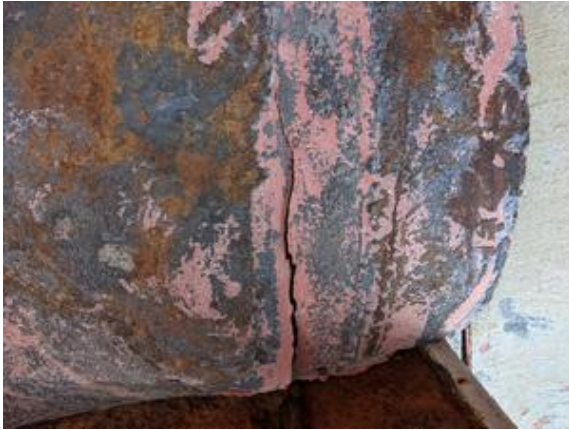
CHE-SP7077-170821-028 thru 030, 1.75% Asbestos, Black/gray subflooring
