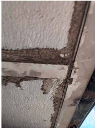
CHE-CNW11111-150721-004 thru 006, Asbestos Not Detected, White/gray sealant
