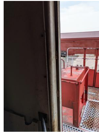
CHE-MP13835-130721-019 thru 021, 4.8% Asbestos, Gray door sealant
