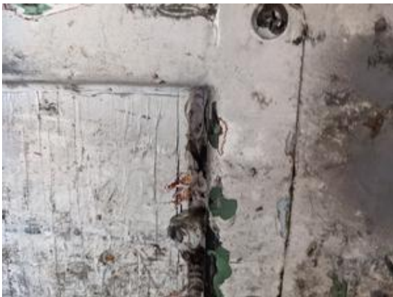
CHE-FTSX812-140721-007 thru 009, Asbestos Not Detected, White sealant
