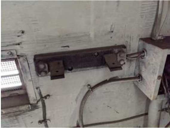
CHE-DRGW01481-160721-010 thru 012, 6% Asbestos, Black Bakelite
