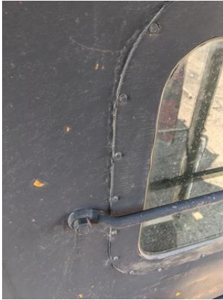
CHE-DRGW01486-160721-001 thru 003, Asbestos Not Detected, Black window caulk
