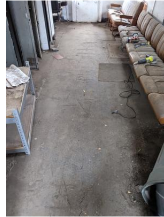
CHE-FTSX812-140721-001 thru 003, Asbestos Not Detected, Black rubberized flooring and clear mastic
