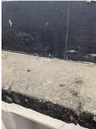
CHE-DRGW01481-160721-013 thru 015, Asbestos Not Detected, Black mastic
