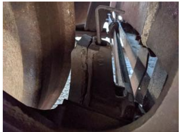
CHE-SP4641-130721-025 thru 027, Asbestos Not Detected, Black Brake Pads
