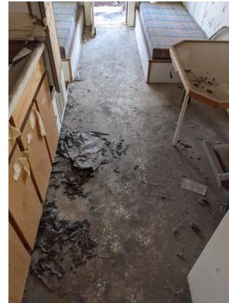
CHE-DRGW01481-160721-004 thru 006, Asbestos Not Detected, White sheet flooring and yellow mastic
