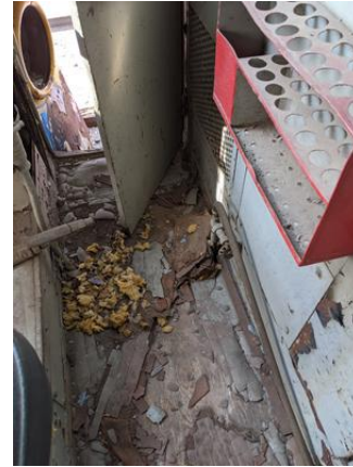
CHE-UP928-160821-037 thru 039, Asbestos Not Detected, Brown Vinyl Flooring (no mastic)
