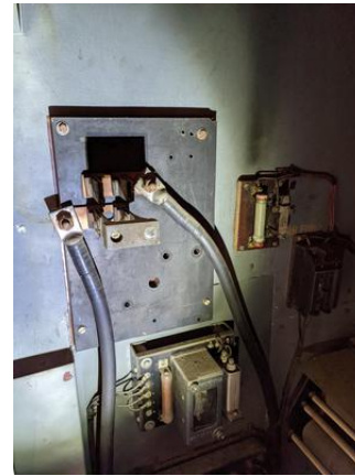
CHE-SP7077-170821-037 thru 039, 20% Asbestos, Gray fireboard
