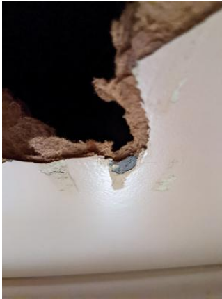
CHE-SP7078-180821-037 thru 039, Asbestos Not Detected, Masonite board (layered compound, mastic and fiberboard)
