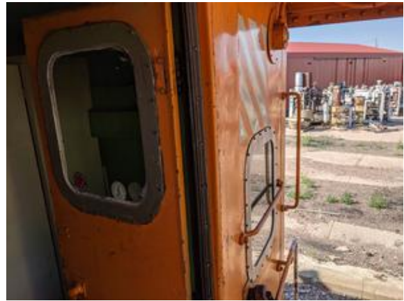
CHE-DRGW01476-170721-001 thru 003, 6% Asbestos, Gray/black window caulk
