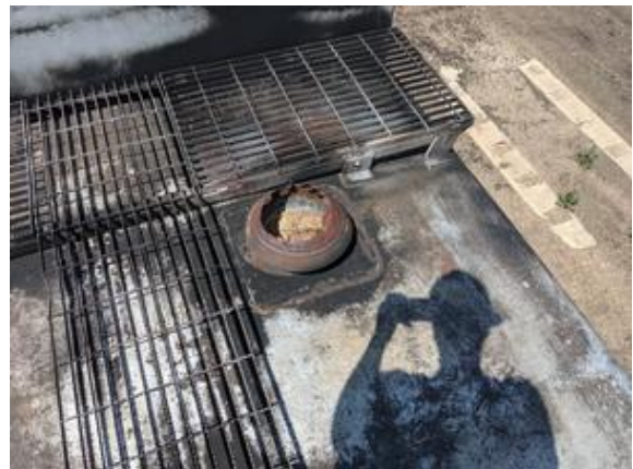
CHE-DRGW01486-160721-007 thru 009, 8% Asbestos, Brown/white sealant
