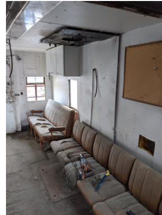
CHE-FTSX812-140721-004 thru 006, 15% Asbestos, Gray transite
