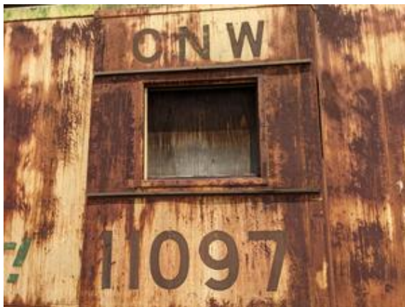
CHE-CNW11097-140721-002L, 0.014% Lead, Yellow
