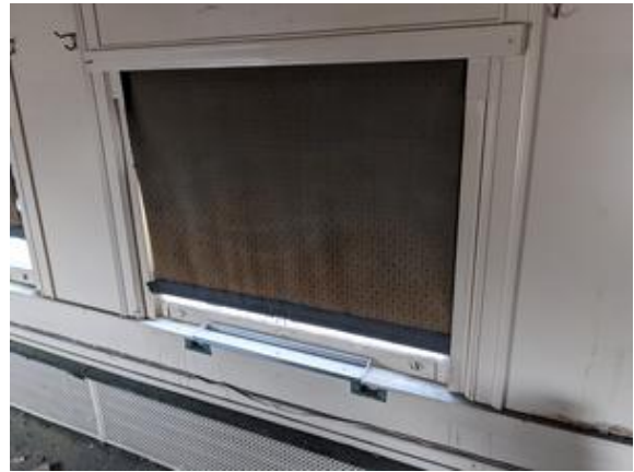
CHE-SP7078-180821-034 thru 036, Asbestos Not Detected, Silver coating
