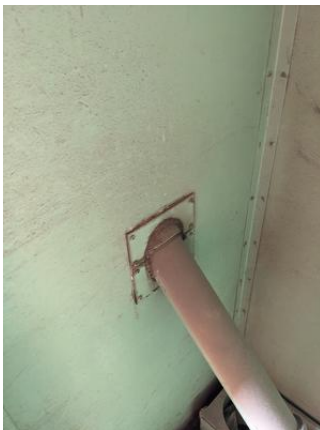
CHE-SP4641-130721-022 thru 024, 10% Asbestos, Gray oil tank sealant
