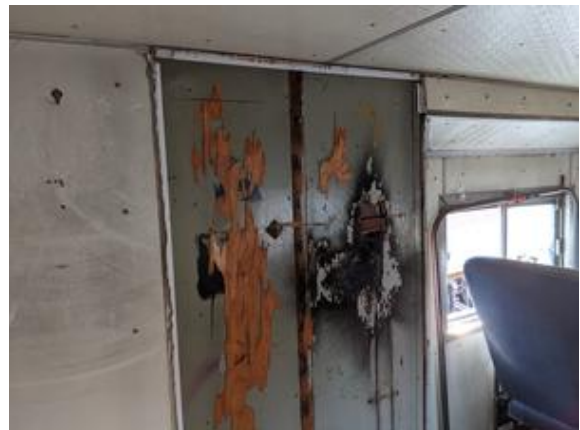
CHE-CNW11111-150721-007 thru 009, Asbestos Not Detected, Yellow mastic
