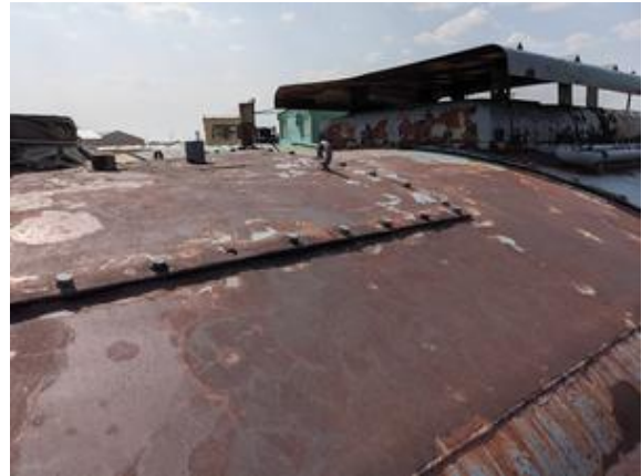
CHE-UP928-160821-031 thru 033, 10% Asbestos, Gray Coating
