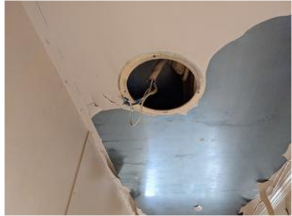
CHE-SP7077-170821-025 thru 027, Asbestos Not Detected, Black/brown electrical wire coating
