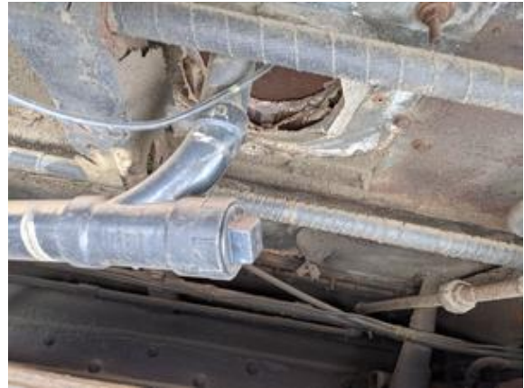
CHE-SP7077-170821-019 thru 021, 2.2% Asbestos, Gray sealant
