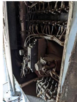
CHE-UP928-160821-016 thru 018, Asbestos Not Detected, Gray Bakelite
