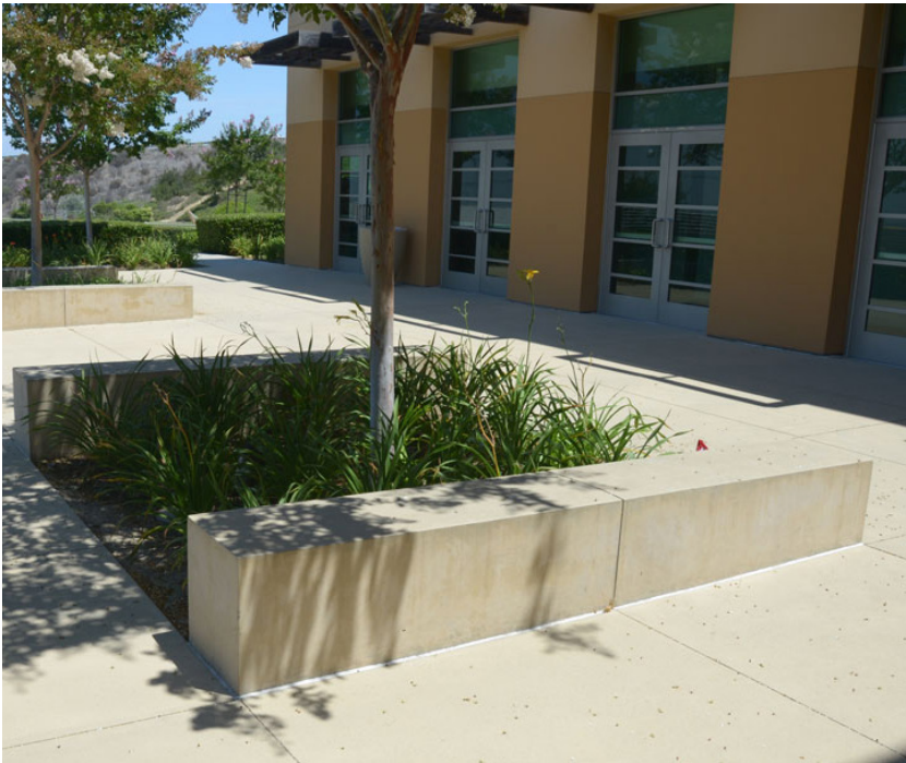
Cast-in-place Concrete Bench
