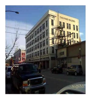
"The Hynds Building incorporated an enormously advanced design for its time. The structure has no interior or exterior supporting walls. Its mass is carried on a steel 'I' beam frame, with poured concrete ceilings and floors. In keeping with Mr. Hynds' wish that the building be fireproof, no wood was used in its construction. All doors, casings, windows, and frames are metal, as is even the decorative picture rail.
