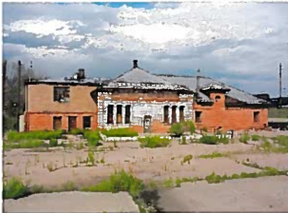
Photo #1 West Elevation
