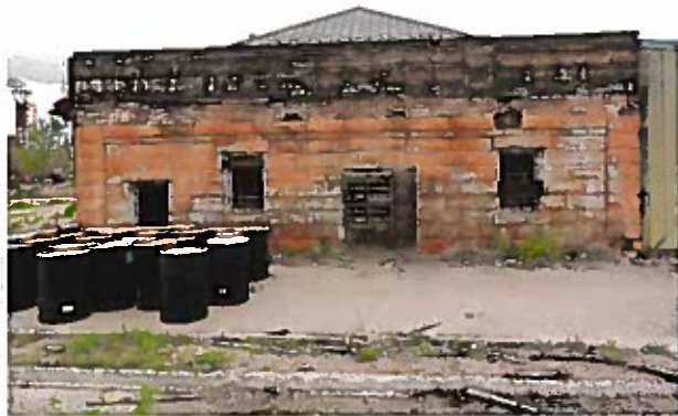
Photo #2 South Elevation
