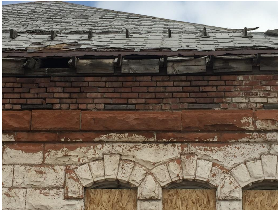
Figure 5 Note metal shingles under asphalt shingles.
