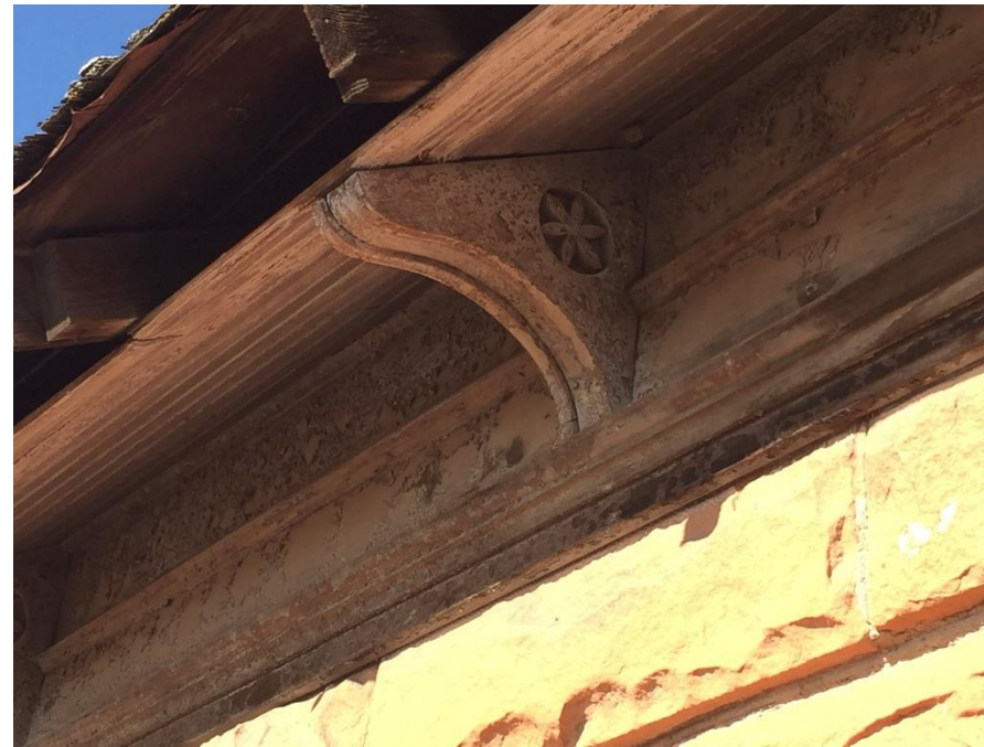
Figure 4 Frieze and bracket detail.
